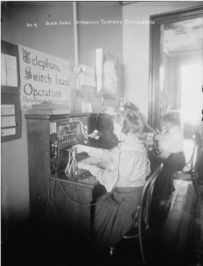
Women working at manual switches would dress neatly as was in keeping with their task of not only efficiently transferring calls but also providing polite personal service to callers. "Women switchboard operators." Courtesy of the Library of Congress.
