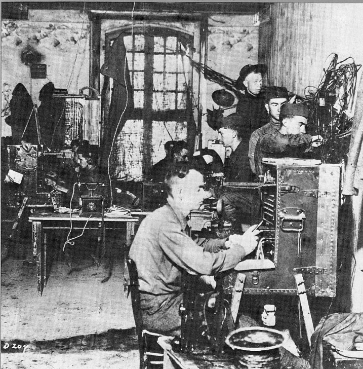
In France during World War I, vital messages were switched over this WE "Camp" switchboard, one of many special products we made for the armed services.
