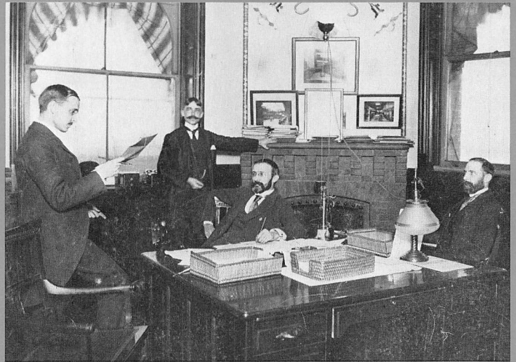
This is the front office at our New York factory at Thames and Greenwich Streets about 1893. Left to Right, A. L. Salt, later president of Graybar; C. E. Scribner, later chief engineer; H. B. Thayer, later president of Western Electric and AT&T; and H. M. Sage, assistant manager and later manager at Clinton Street in Chicago.
