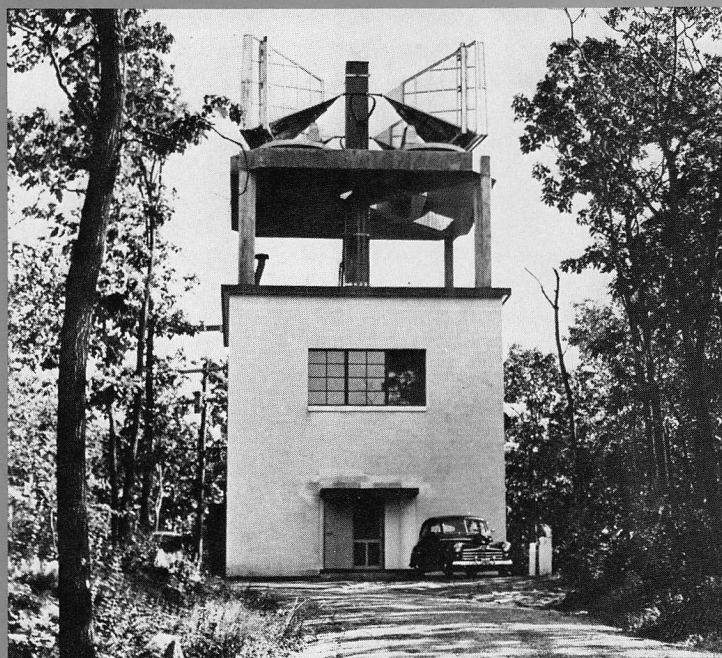
One of the very first microwave radio repeater stations on the route between New York and Boston. This photo is dated November 13, 1947. Very quickly microwave became the backbone of the long distance telecommunications network.
