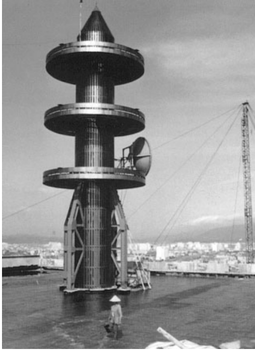
Figure 25.17 Radio-relay tower in Taipei, Taiwan-China, 1973. (Courtesy of Alcatel SEL.)
