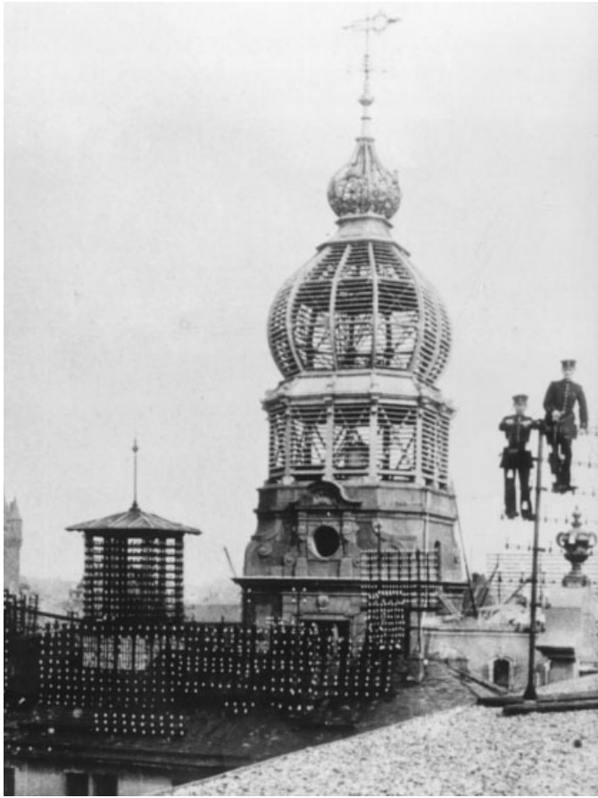
Figure 20.2 Open-wire support and access tower on the roof of a telephone exchange. (Courtesy of Museum für Kommunikation, Frankfurt, Germany.)
