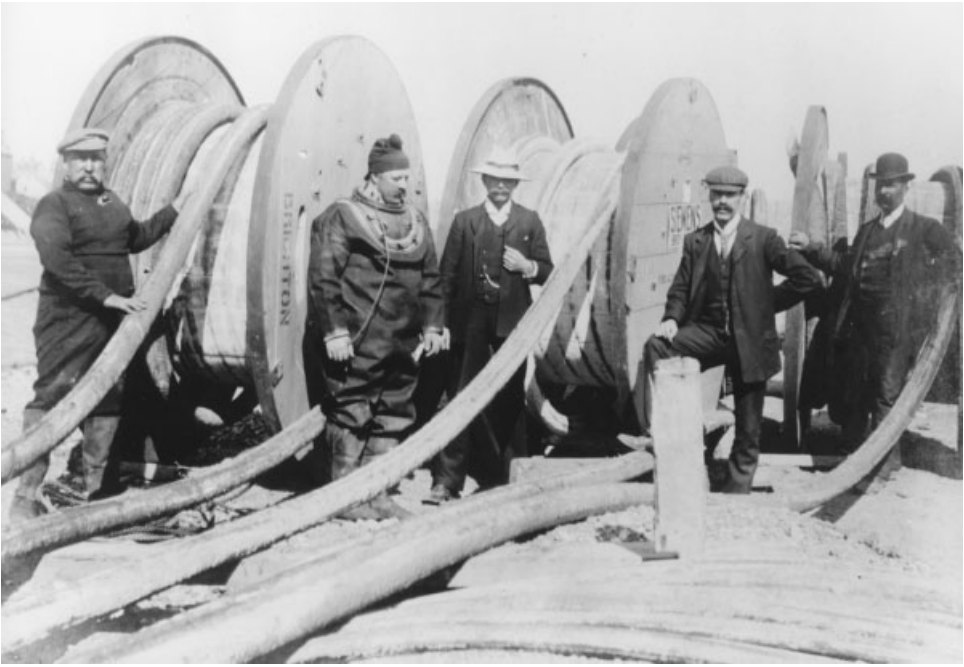
Figure 8.22 Transatlantic cable at the factory. (Courtesy of Siemens Press Photo.)
