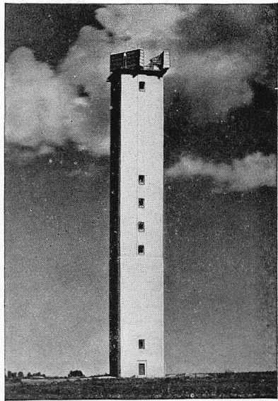
This 200-foot tower is part of the radio relay system that beams telephone calls and television programs across the nation.
