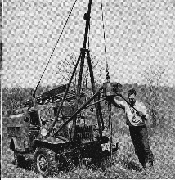
Power driven augers, as pictured above, help speed the construction of rural telephone lines. At left: Linemen string wires to serve more farm telephones.
