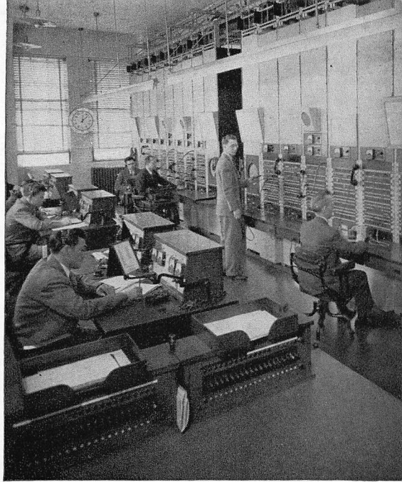
Long Lines control board and equipment for setting up radio broadcasting networks for transmission of programs over special telephone channels.
