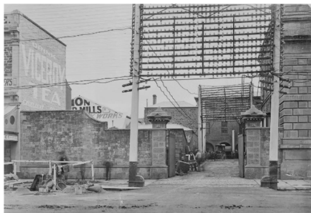
View to rear yard from Franklin Street following construction of 1893 wing Note distant three-level brick building opposite gateway (1893) and original perimeter wall and gates
