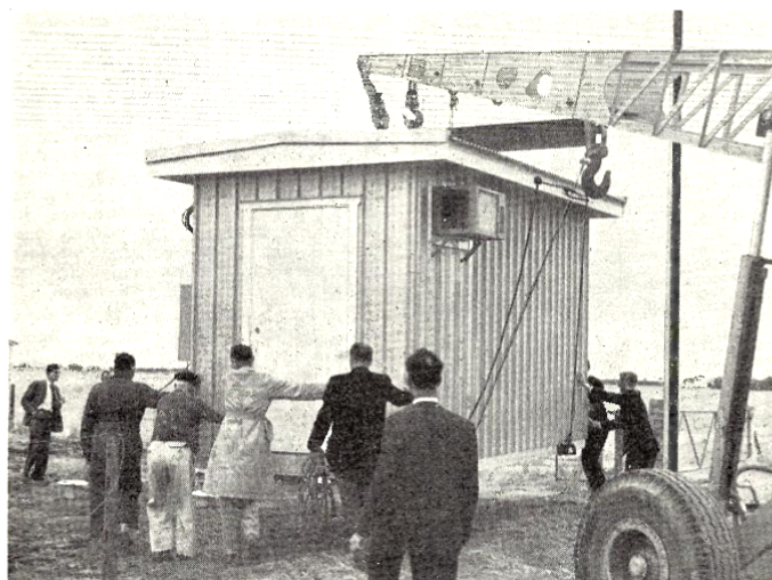
Fig. 10.—Reeves Plains ARK 511 Portable Exchange.
