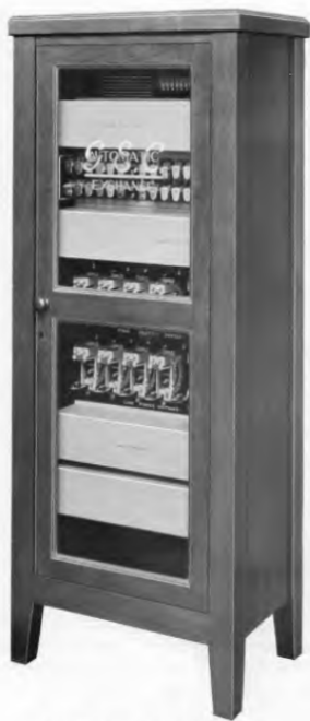
Fig. 2.—Typical 24-line non-extensible R.A.X. (Ref. No. 9071).
