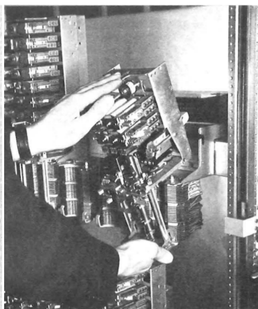
— JACKING-IN A SELECTOR.
